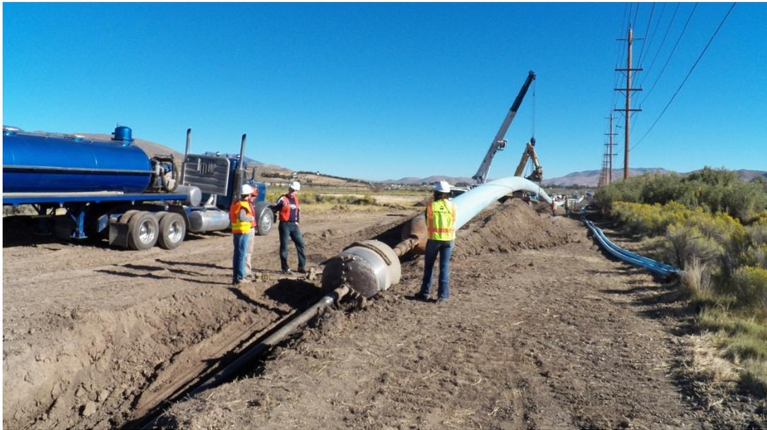
**FIGURE 3-12. INTERCONNECTING TWO WATER SYSTEMS**
