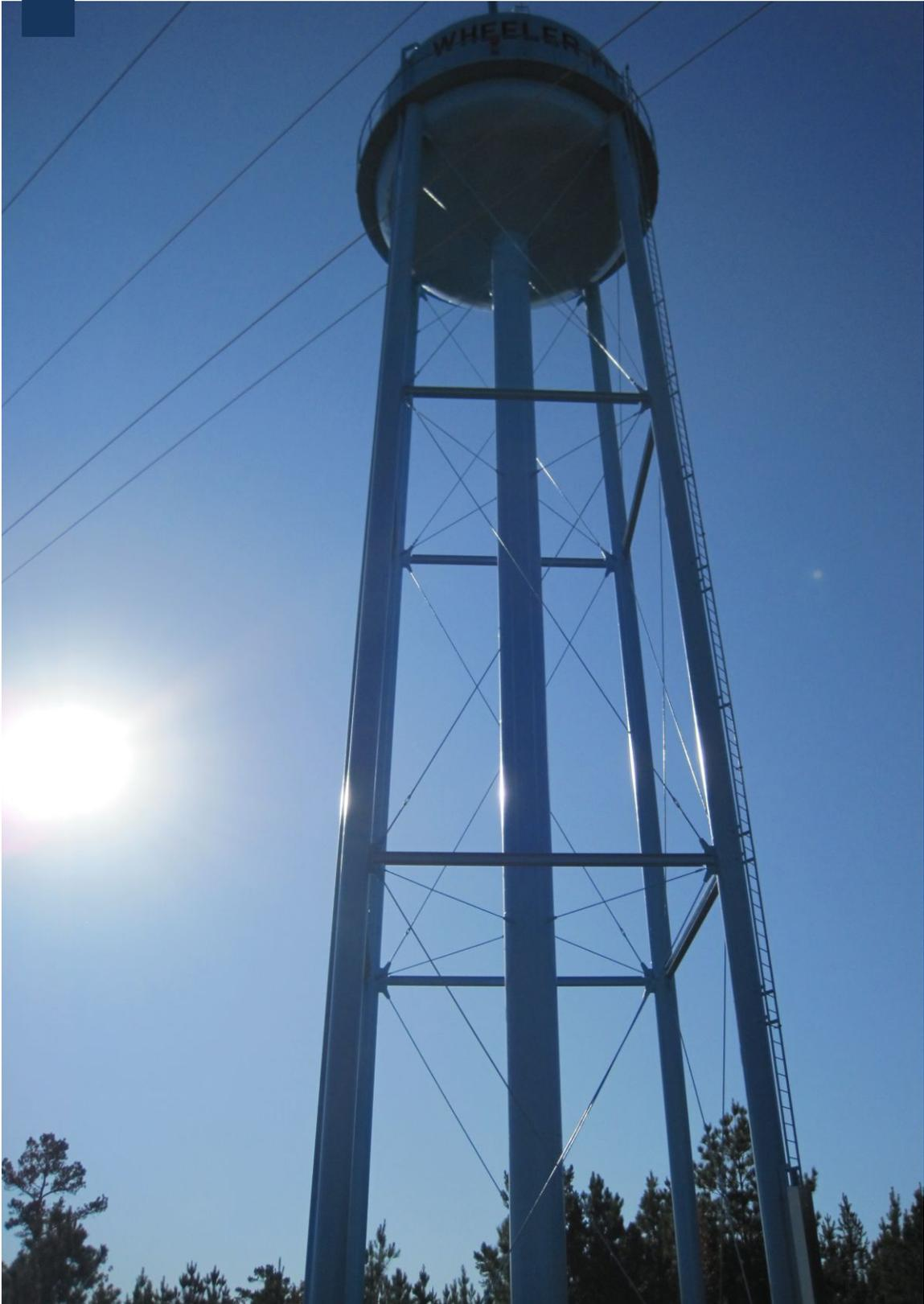
*In order to ensure public health is protected, this newly installed 100,000 gallon elevated storage tank must be properly maintained by the water system with oversight by the state drinking water program staff.
