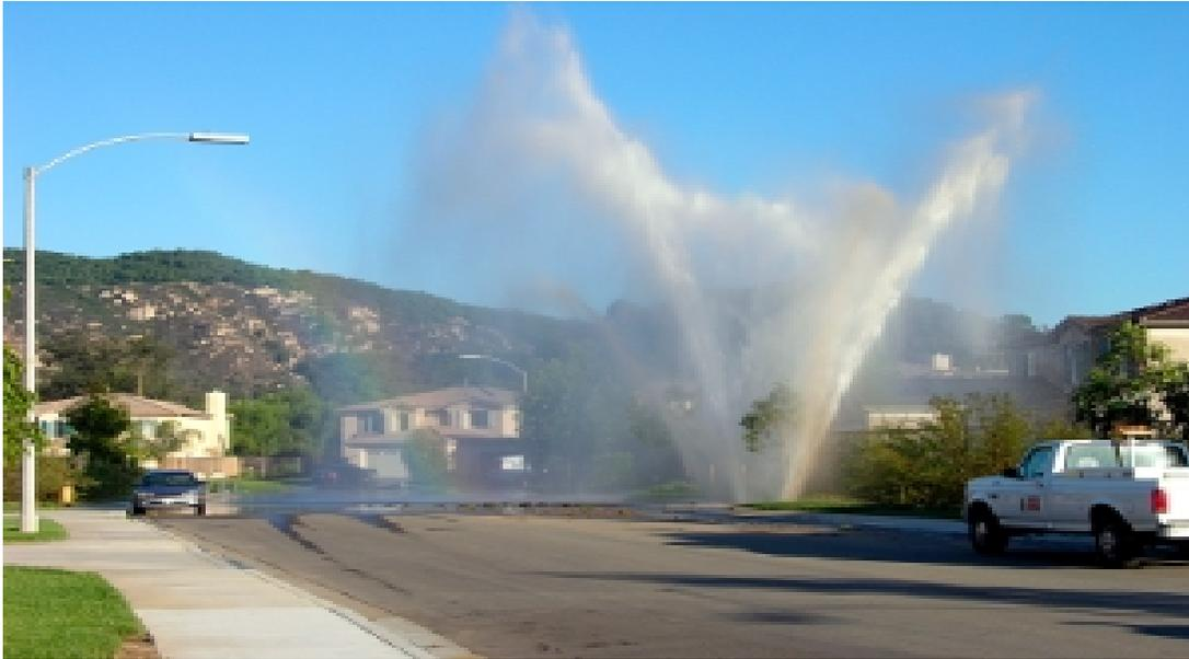
**FIGURE 3-11. RUPTURE OF A 66-INCH WATER MAIN**
