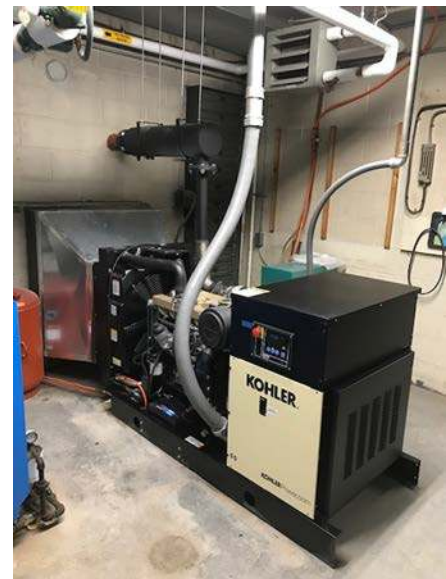
Eureka Water Treatment Plant
