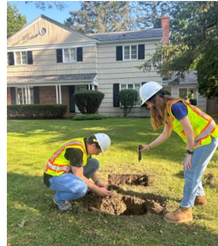
Paired inspections with normal operations
